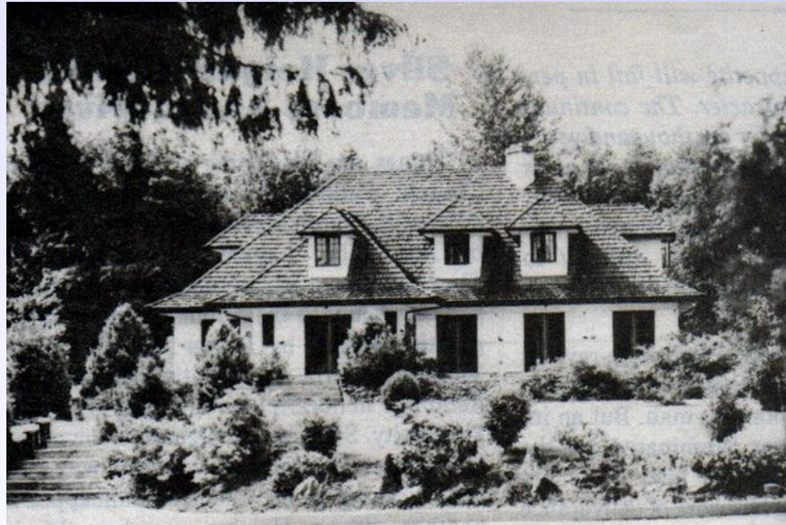
Radiant Living Evangelistic Centre for Metropolitan Vancouver.
